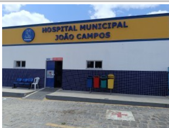
Vista Frontal do Hospital
